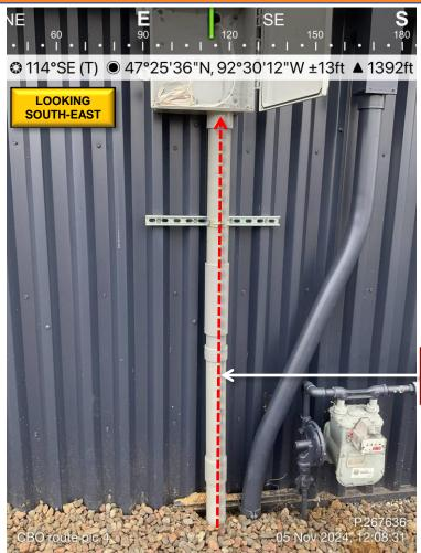
**LUMEN TO: PULL 175FT OF NEW 24CT FIBER** THROUGH EX. CBO FROM CUST HH (17+95) **TO MPOP ENTRY (19+70).**
