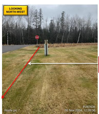
**LUMEN TO: BORE & PLACE 850FT OF NEW** 1.25IN CONDUIT & PULL NEW 24CT FIBER FROM HH-4280 MILLER TRUNK RD-2 (09+45) TO CUST HH (17+95).
